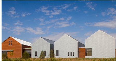
Harriet Tubman Underground Railroad Visitor Center Cambridge, MD
