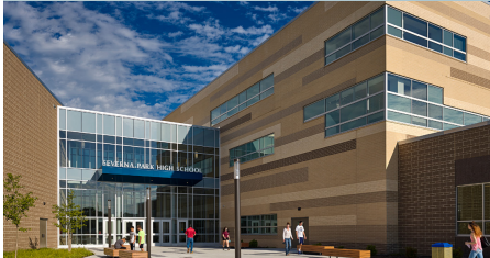
Severna Park High School Severna Park, MD
